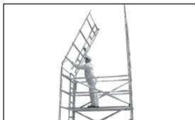
14 Continue erecting tower to final tower height repeating the process as illustrated. Always ensure that there is side protection to prevent falls. Maximum vertical distance between platforms must not exceed 4m.
