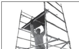
15 Remove plain platform from the bottom and reposition as shown.
