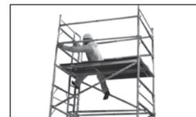
19 Dismantling is the reverse except when dismantling the handrails. Undo the four end hooks and from the sitting position remove the handrails. Do not remove the handrails whilst standing on the platform, this would leave you at risk.
