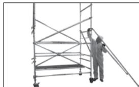
11 Secure stabilisers as soon as possible to increase tower stability. Check tower kit list to ensure the correct stabilisers are fitted.
