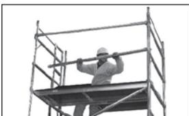
17 From the sitting position through the trapdoor, fit four handrail braces to vertical member of frames.
