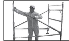
4 Klik in diagonal braces, starting at the bottom rung. Braces should be added in a continuous pattern. When fitting a full intermediate work platform it is permissible to interrupt the continuous pattern.
