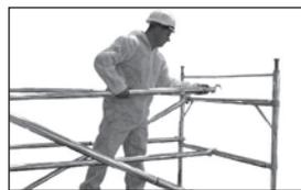
7 Fit four handrail braces, two on outside and two on mid rung of frame as shown, on lower levels these may not be required.
