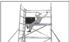
13 From the sitting position through the trapdoor, fit four handrail braces, two on the outside and two on the inside as shown.
